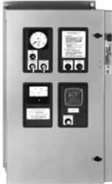
Wall-Mounted C-HRG (resistors not shown)
