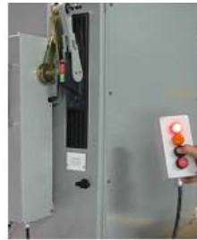
Ampgard MV Starter ISO Switch Operator
