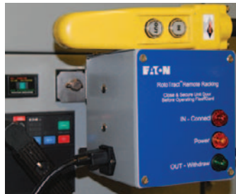
FlashGard LV MCC Remote Racking Device
