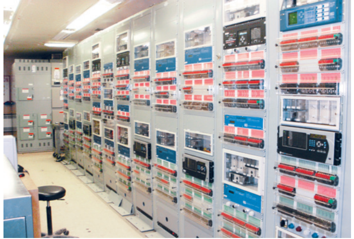
Station following completion of electrical upgrades
