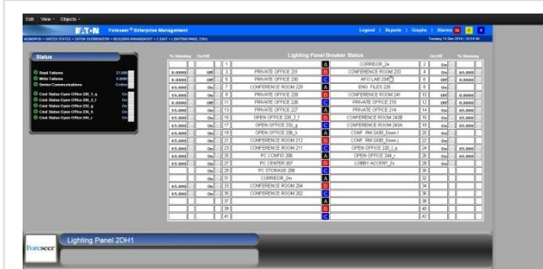
Branch circuit monitor
