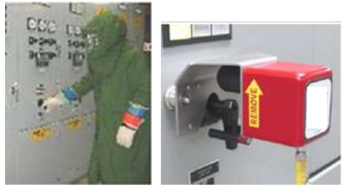
Figure 12. Local switching (Left) vs. Remote switching (Right)
