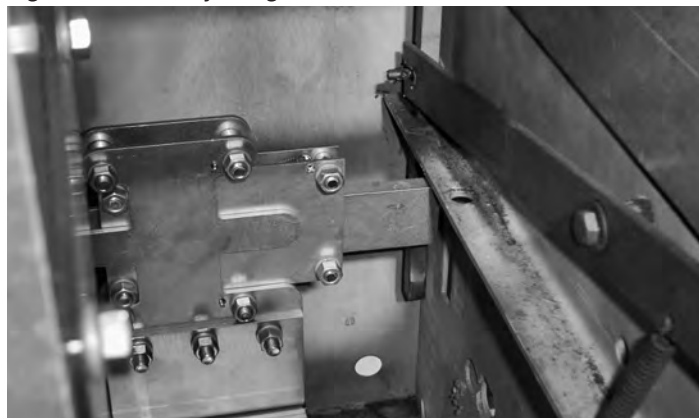
Figure 5.8. Self-Adjusting Anti-Rotation Device
