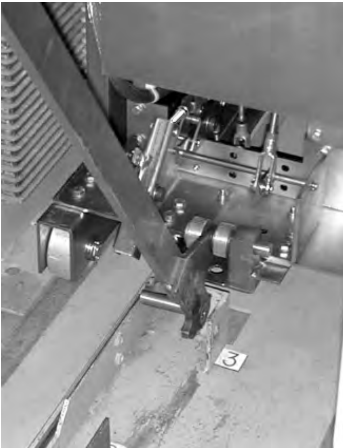
Figure A.2. Rack-Out Position of Levering Handle
