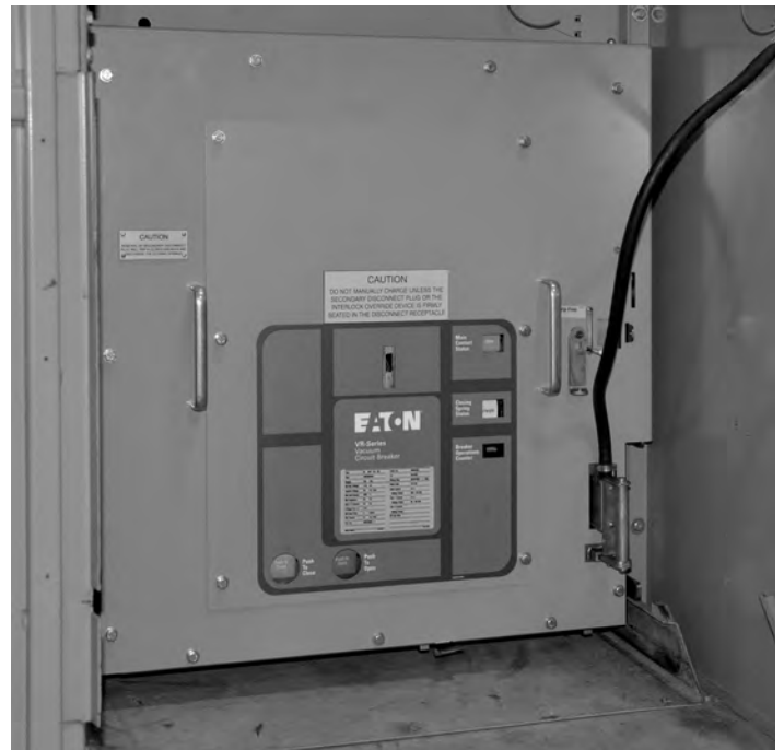
Figure 5.8. 15PV-VR in the Connect Position (1200A Shown)
