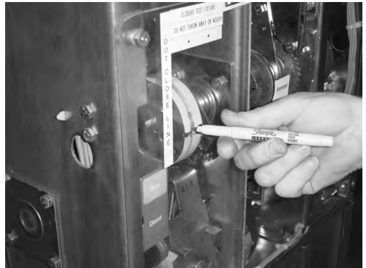
Figure 6.12. Move the Sharpie® 15° Left and Right
