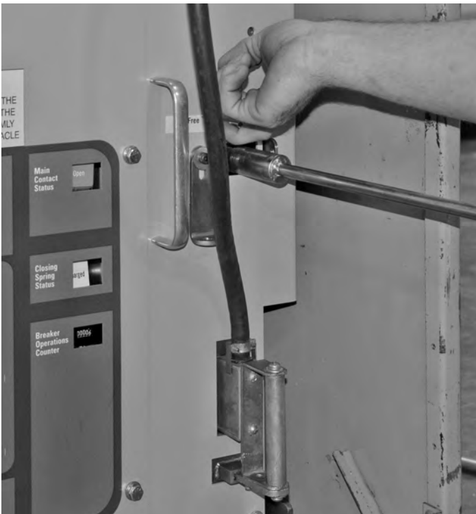
Figure 5.7. Racking Handle Engagement
