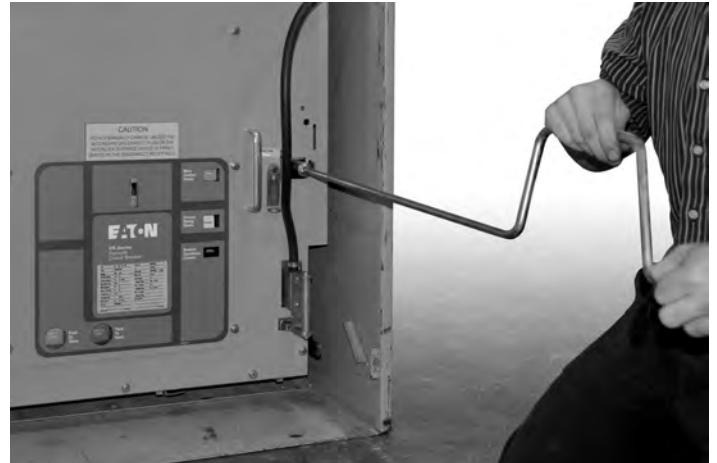
Figure 5.8. Racking Into Cell (15PV-VR 1200A Shown)
