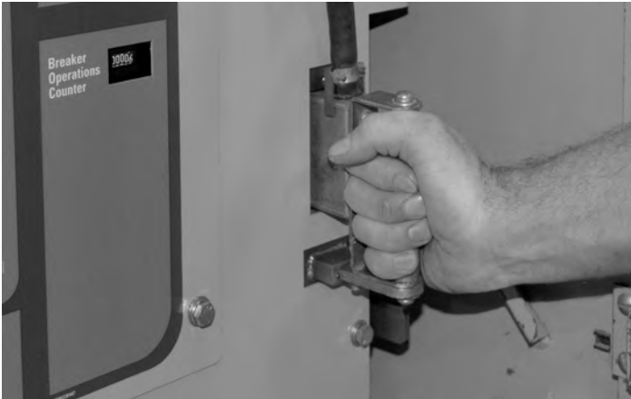
Figure 5.6. Manually Plugging Secondary Disconnect
