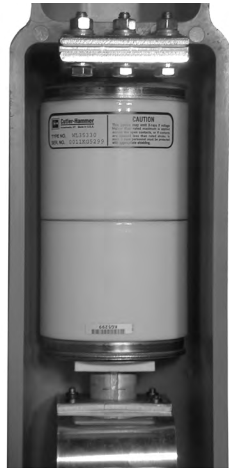
Figure 4.1 5/15PV-VR Interrupter Assembly (18WR Design Shown)
