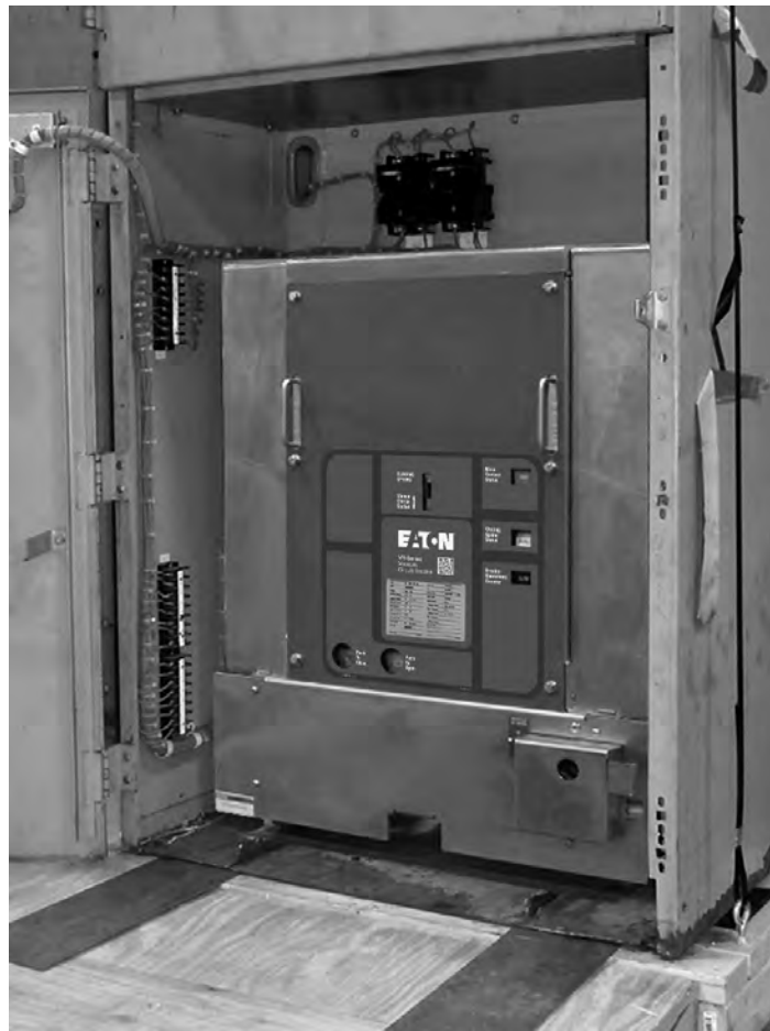
Figure 5.4. 15VHK-VR Model 20 in the Disconnect Position
