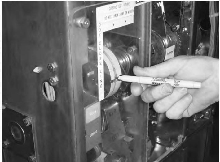
Figure 6.12. Move the Sharpie® 15° Left and Right
