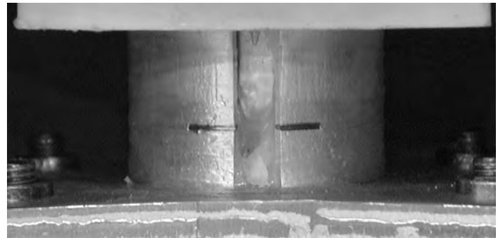
Figure 6.1. Vacuum Interrupter Showing Contact Erosion Indicator With Breaker Open (Shown here for clarity purposes only)
