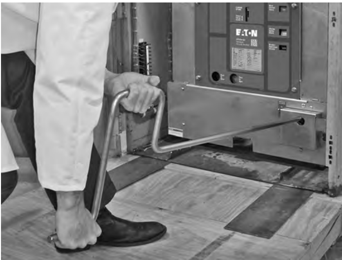
Figure 5.5. Racking Handle Engagement (1200A Shown)
