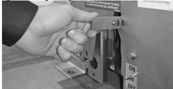
Figure 5.8. Lifting Racking Access Handle
