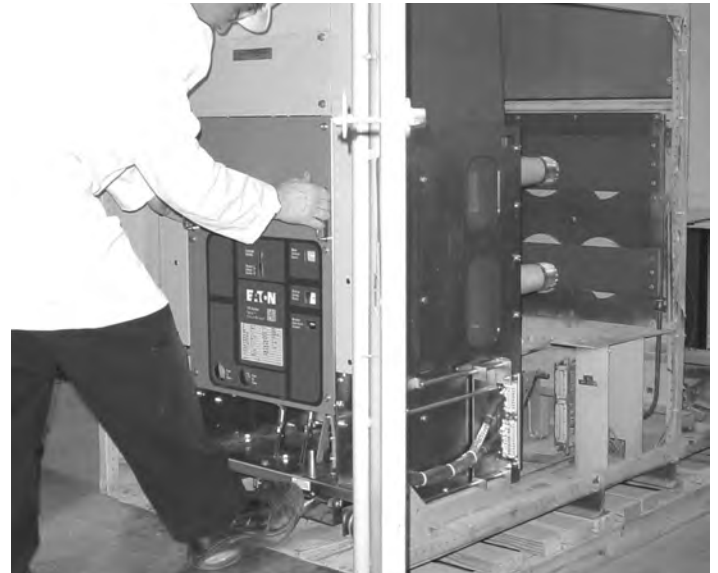
Figure 5.4. Insertion of DST-2-75-VR
