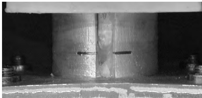
Figure 6.1. Vacuum Interrupter Showing Contact Erosion Indicator With Breaker Open (Shown here for clarity purposes only)
