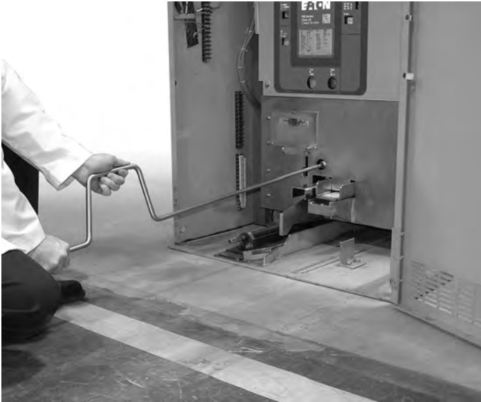
Figure 5.19. Inserting FC-VR with Internal Rotary Racking
