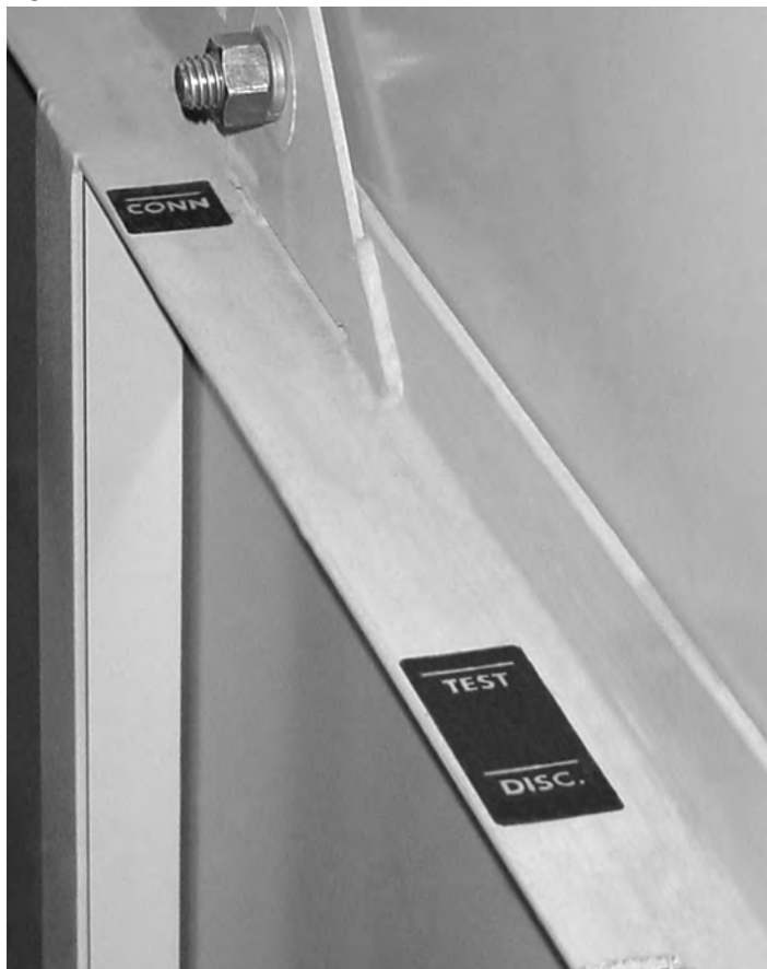
Figure 5.13. Cell Position Label Detail
