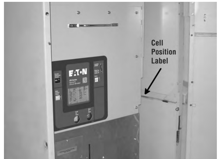
Figure 5.12. Cell Position Label Location
