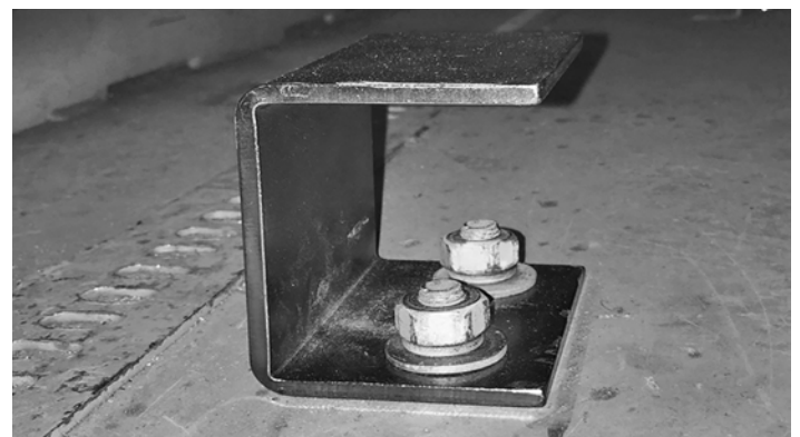
Figure 5.4. FC-VRG Code Plate Mounted in Switchgear Structure
