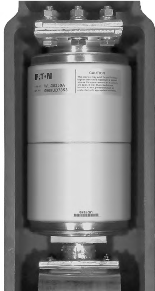
Figure 4.1. 18WR Interrupter Assembly
