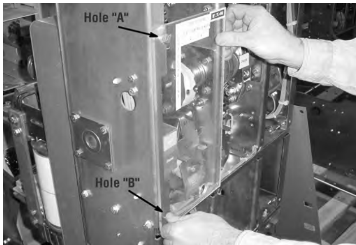
Figure 6.7. Attaching CloSure™ Test Tool at Hole "A" & "B"
