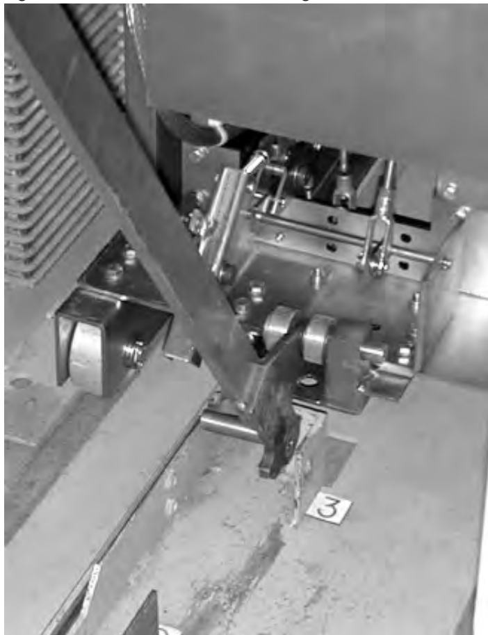
Figure A.2. Rack-Out Position of Levering Handle
