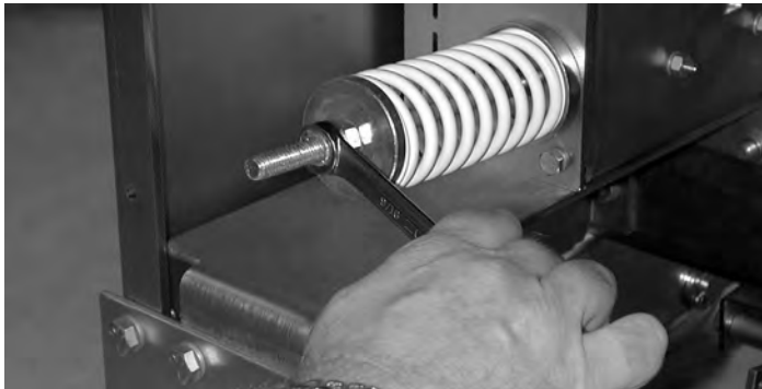
Figure 5.5. SURE CLOSE Spring Compression Setting
