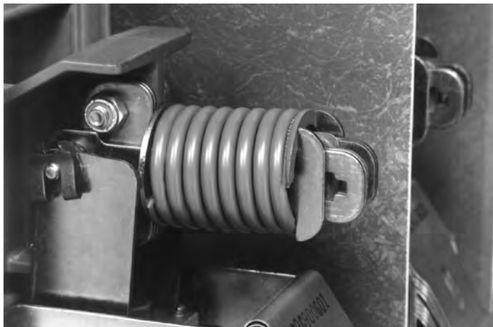
Figure 6.3. The Arrow Shows The “T” Contact Wipe Indicator - Example with Blue Spring (If the “T” or any portion of its visible as shown with the breaker closed, the wipe is satisfactory) (See Next Figure for Graphic of All Possibilities)
