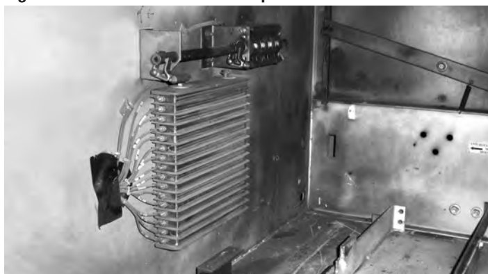
Figure 5.3.b. Cell Mounted MOC Operator
