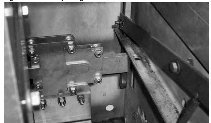
Figure 5.8. Self-Adjusting Anti-Rotation Device
