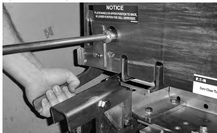
Figure 5.10. Racking Access Handle
