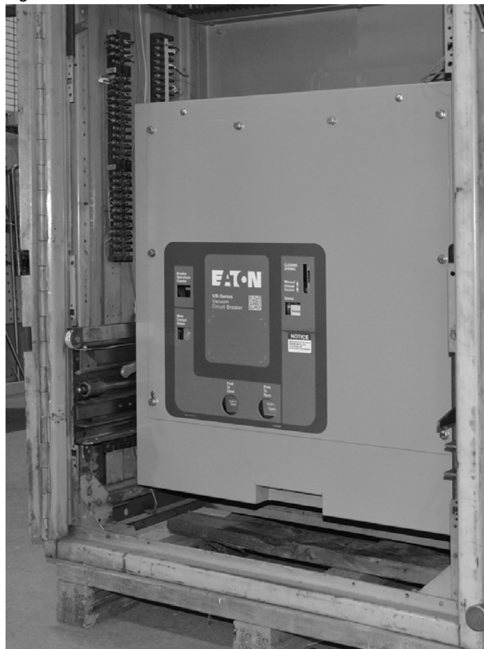
Figure 5.4. VB1-VR in the TEST Position
