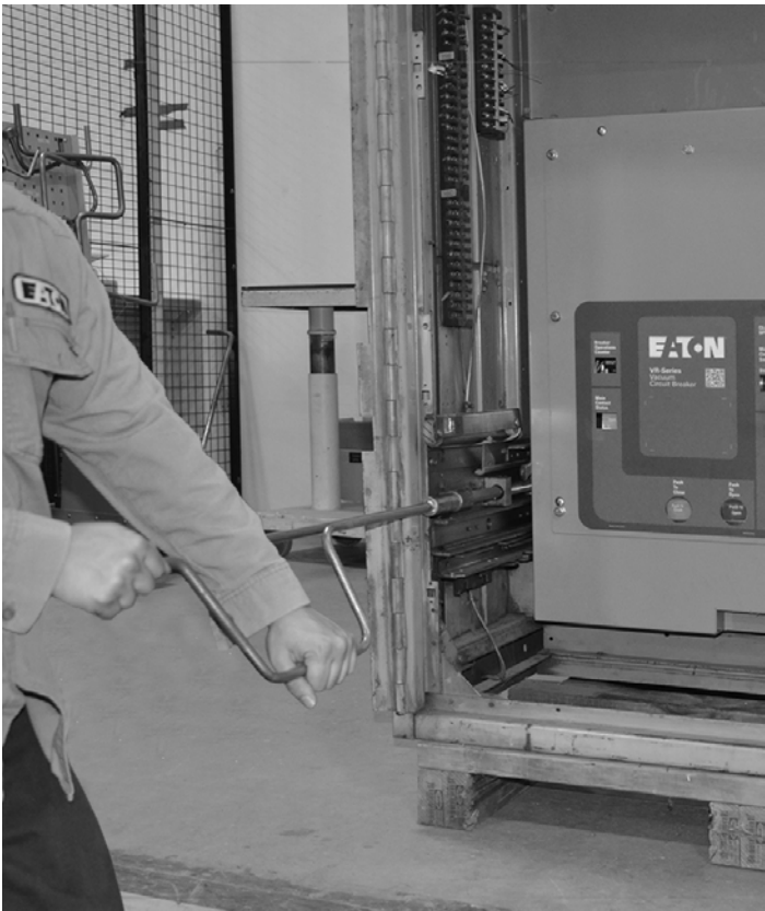
Figure 5.5. Racking Handle Engagement (1200A Shown)
