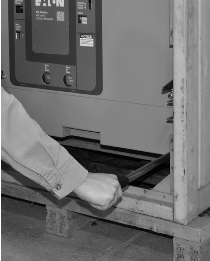
Figure 5.6. Engagement of Secondary Disconnect
