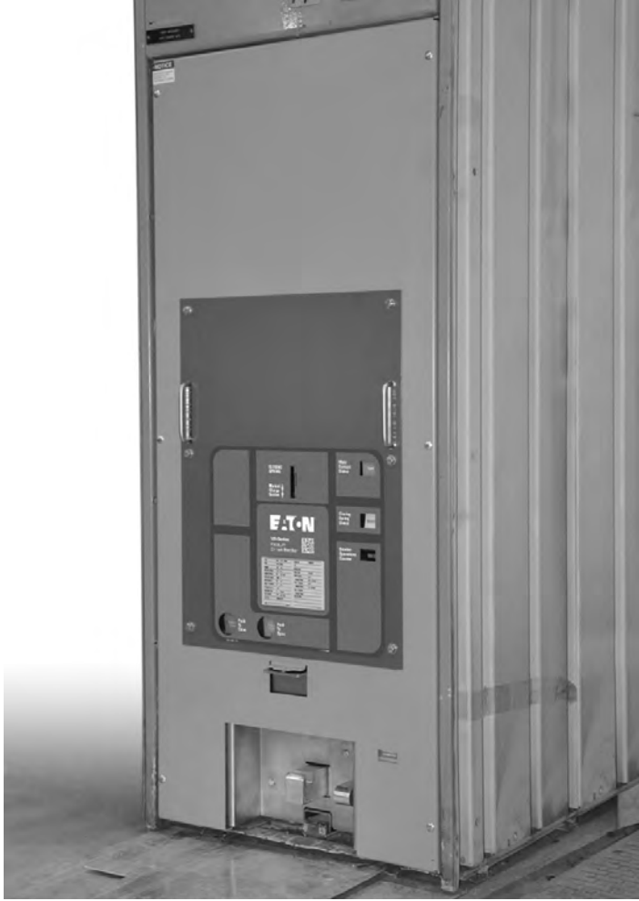
Figure 5.6. AMH-VR in the Connect Position
