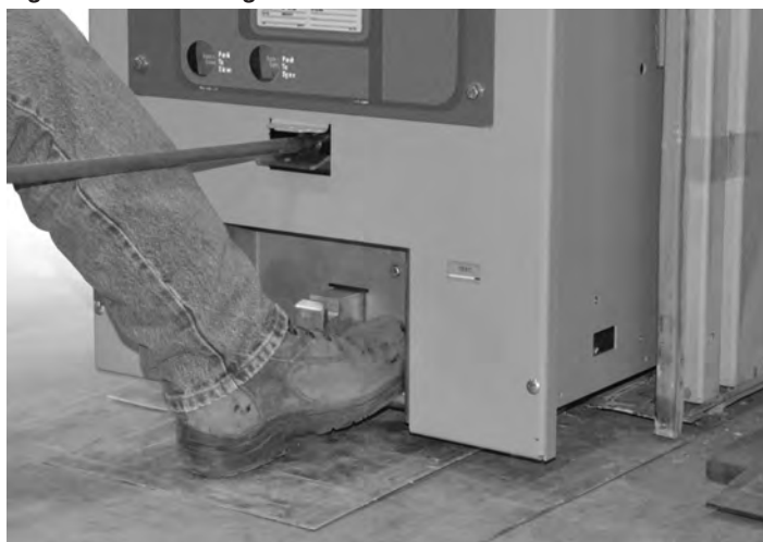
Figure 5.3. Advancing the AMH-VR Into the Cell
