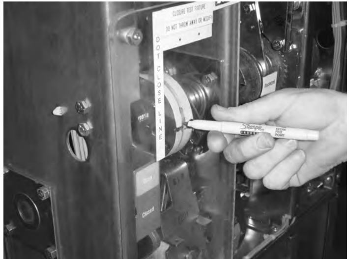
Figure 6.12. Move the Sharpie® 15° Left and Right
