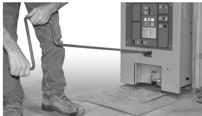
Figure 5.5. Racking the AMH-VR Into the Cell
