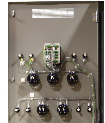
Protective Relaying / Switchgear Door Upgrades
