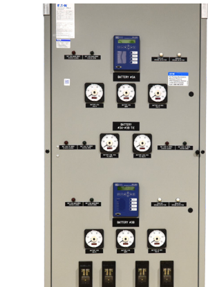
Protective Relaying / Switchgear Door Upgrades
