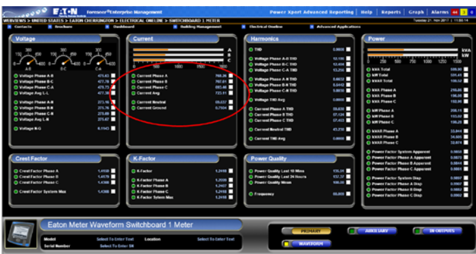
Figure 3. An EPMS can automatically track load levels by phase, giving instant notification when extreme imbalances begin to occur
