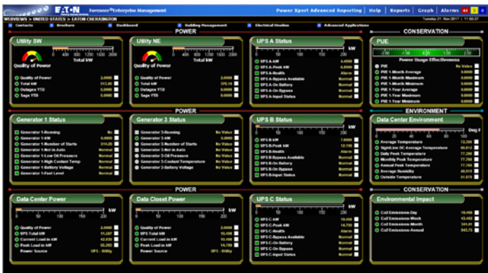
Figure 1. An EPMS system should provide an user-defined overall view of your power consumption
