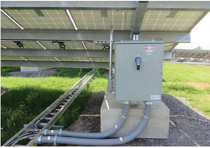
Eaton Crouse-Hinds series DC disconnect and B-Line series cable management system
