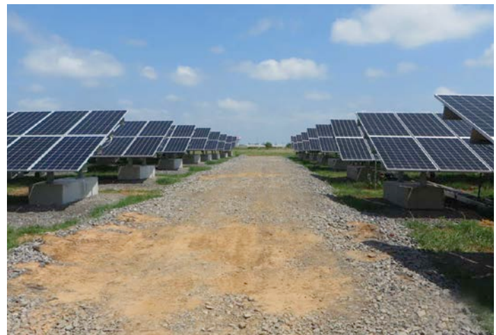
Maintenance access road for Phase I installation
