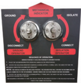
Visible isolation and ground mechanical indicator
