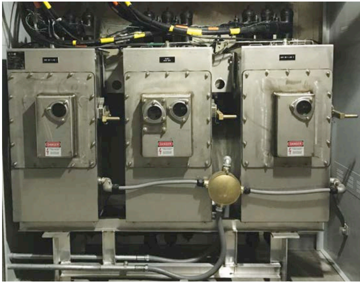
Multi-way VisoVac-CE with remote pushbutton control, SCADA and HMI ready
