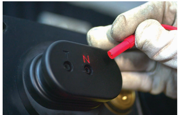
Figure 7 – Phasing test leads installed
