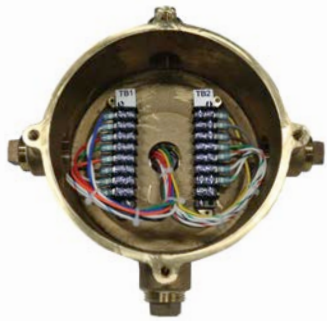
Bulkhead with cover removed
