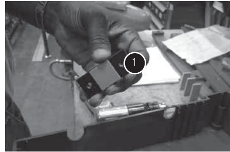
① With Remote Racking removed, peel off tape backing and install brackets on inside of cover. Tighten bolts to secure brackets in place. Leave hardware in.
