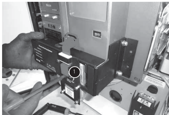
① Slide the Remote Racking in to place and install the mounting hardware.
