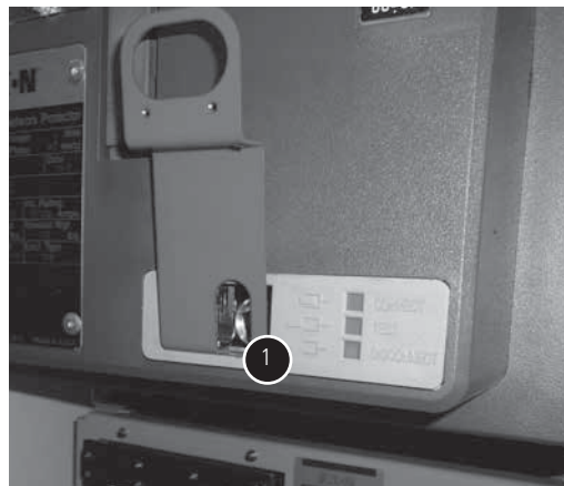
① Slide lifting bracket under shutter.
