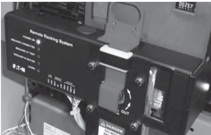
① Remove small cap and depress button start programming. Learn Mode LED will illuminate.
