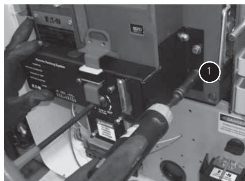
① Tighten the six mounting bolts.
