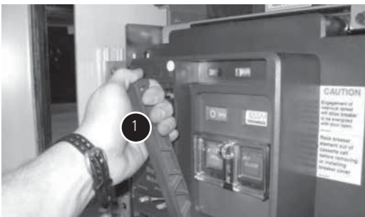
① Crank handle down and pull cover forward to remove.
