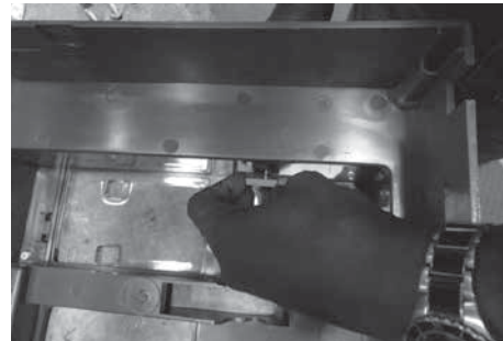
① With Remote Racking removed, peel off tape backing and install brackets on inside of cover. Tighten bolts to secure brackets in place. Leave hardware in.
