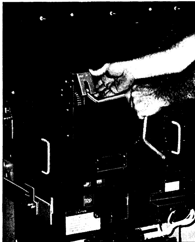
Fig. 6 Inserting Levering Crank Socket Over Head of Levering Shaft
