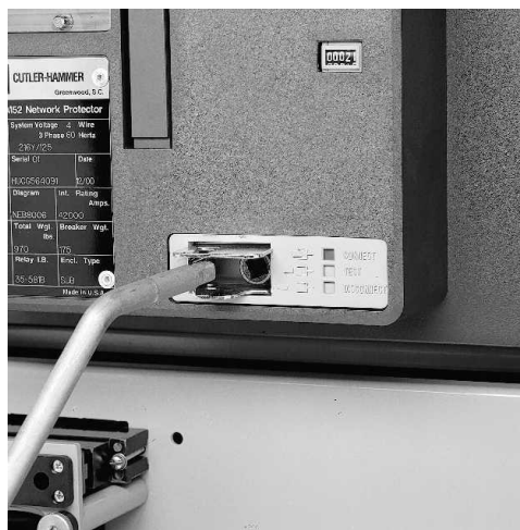
Fig. 7 Inserting Levering -In Crank
