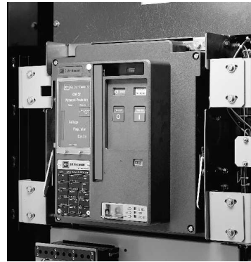
Fig. 8c Breaker in Disconnect Position
