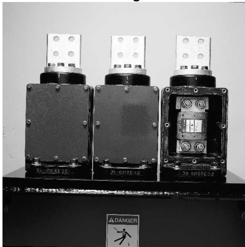
Fig. 3 NPL Fuse Housing (external fuses)
