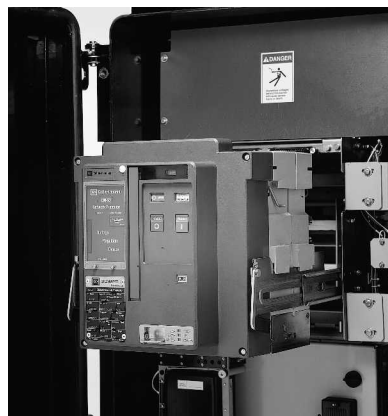
Fig. 10 CM52 w/ Breaker withdrawn
