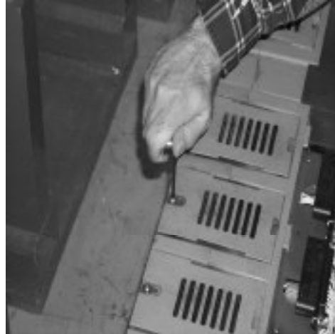
Fig. 13a Loosen Arc Chute captive bolt
