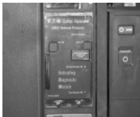
Fig.15 Indicating Diagnostic Module (IDM)
