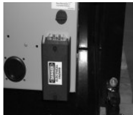
Fig. 17 Test Plug Connector
