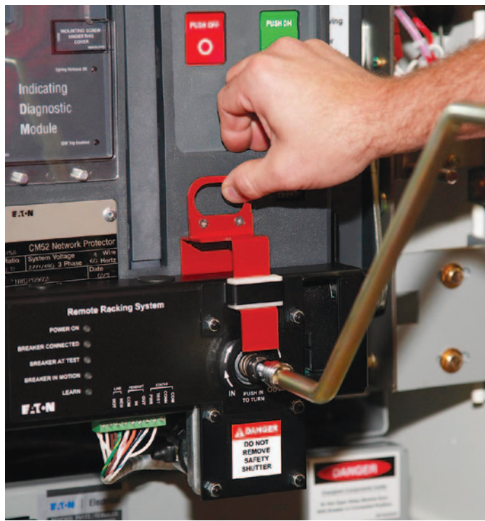
Figure 4. The remote racking unit has a built-in manual crank override under a protective shutter.
