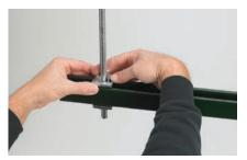
2. Once trapeze is at the desired elevation, snug against the channel by rotating the entire assembly clockwise to a position that is square with the channel (no more than 1/4 turn).
