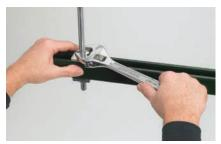
3. To complete assembly, snug hex nut portion of the assembly by turning clockwise against the square washer (4-6 ft-lbs).
