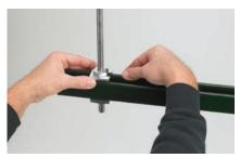
1. Hold Buzznut in open position and install at desired location on ATR. Hand-tighten the hex nut portion of the assembly clockwise to close.
