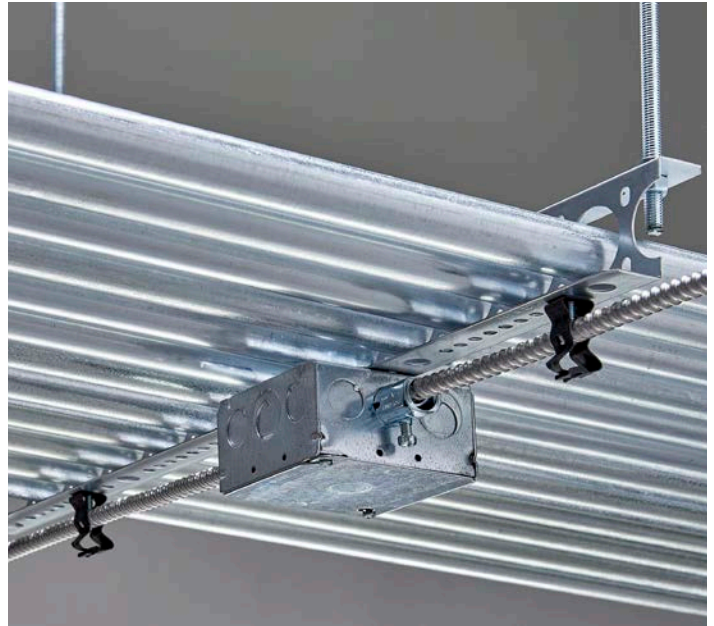
Conduit trapeze support with electrical box
