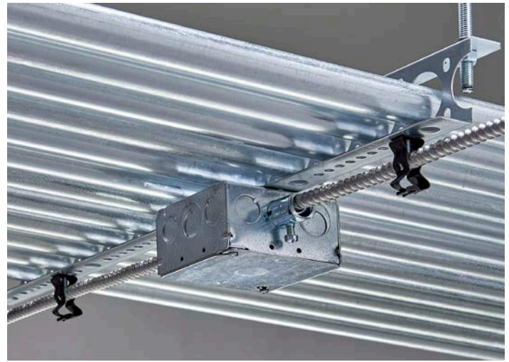
Conduit trapeze support with electrical box
