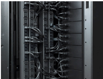
Lacing bars are included for power (ePDU) mounting.
