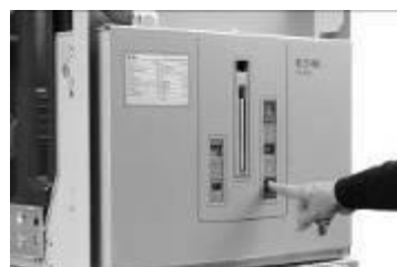
Fig. 5-5: Open manually
