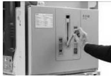
Fig. 5-1: Pull the round handle down
