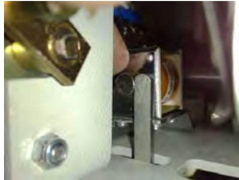
Fig. 5-11A: Cradle Electromagnetic Interlock
