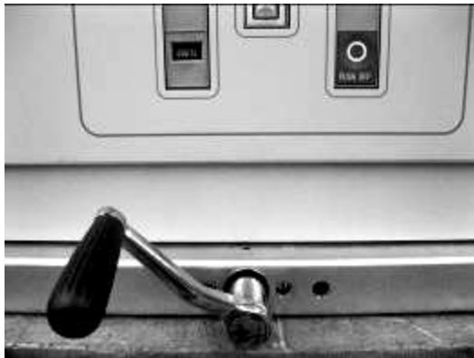
Fig. 5-8: Inserted racking Handle
