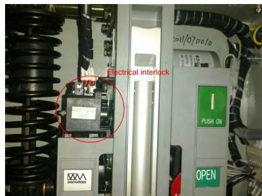
Fig. 5-12B: Mechanism Electromagnetic Interlock
