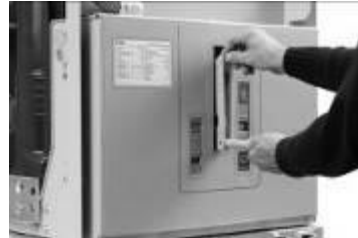
Fig. 5-2: Pull out the handle with two hands
