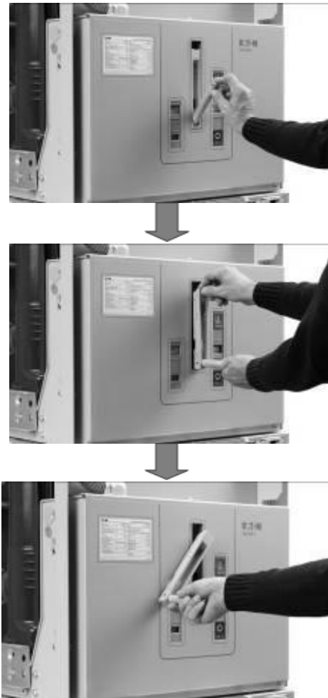
Fig. 6-5: Manual Charging Process
