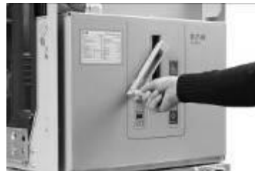
Fig. 5-3: Turn the handle clockwise
