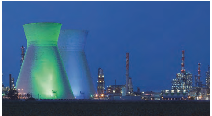
Thermal power station
