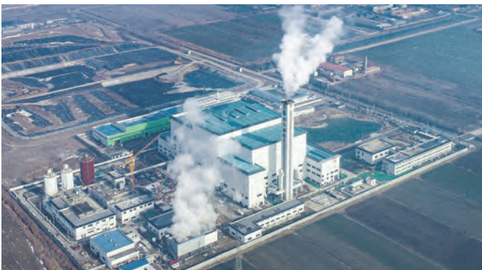
Waste incineration power plant
