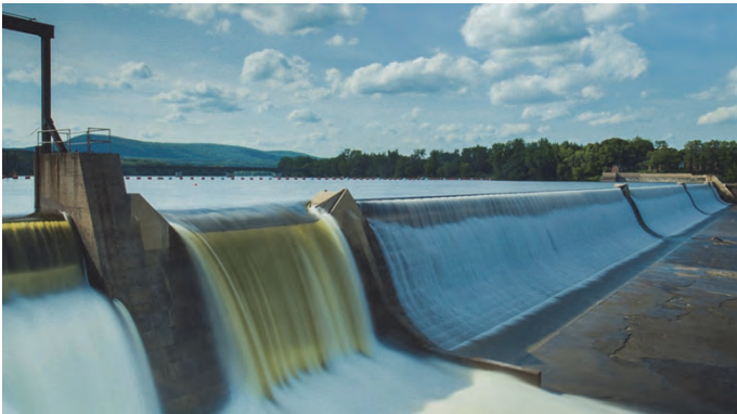
Hydroelectric power station
