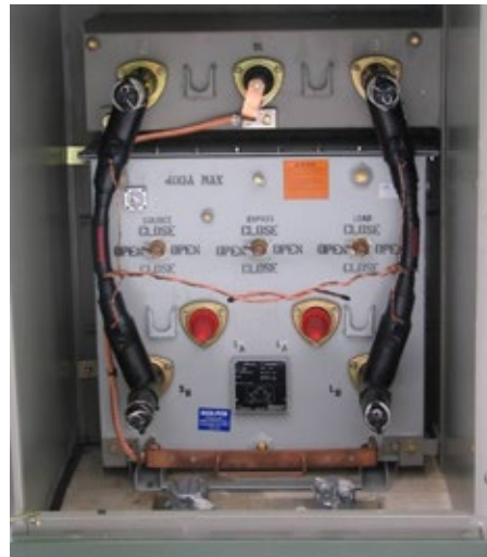
Figure 7. Voltage regulator bypassing operation.
