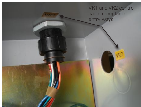
Figure 2. Enclosure entry way examples.
