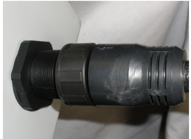
Figure 45. Control cable connected to the GE control box at the bottom.
