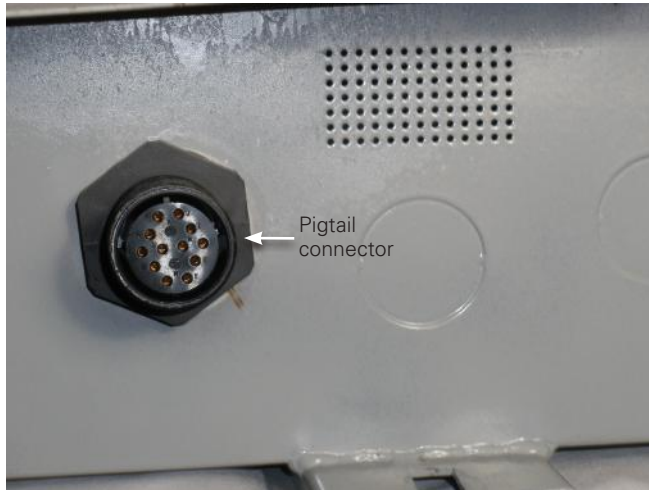
Figure 32. Installation of the pigtail into the bottom of the control box.
