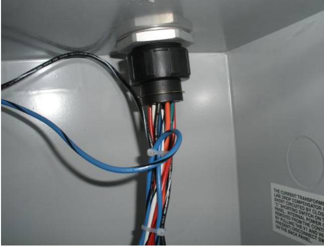
Figure 20. Installed pigtail connector on control cable.
