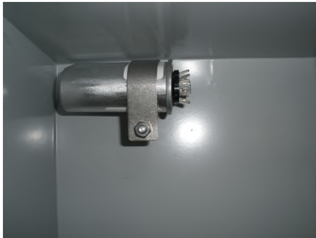
Figure 24. Motor capacitor mounting provision.
