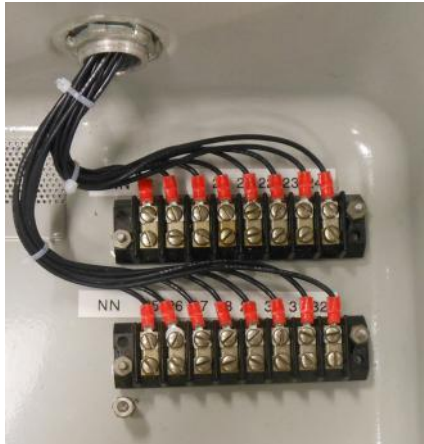
Figure 28. Leave the NN terminal boards and wiring from the regulator into the control box in place.
