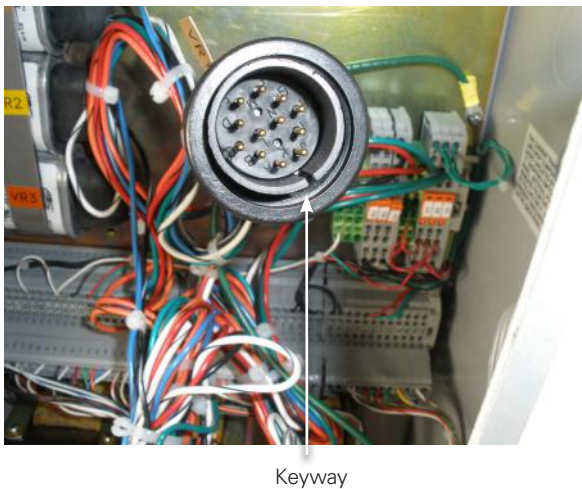
Figure 6. Male pigtail harness connector.
