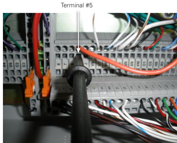
Figure 23. Relocate the orange wire to terminal 5.
