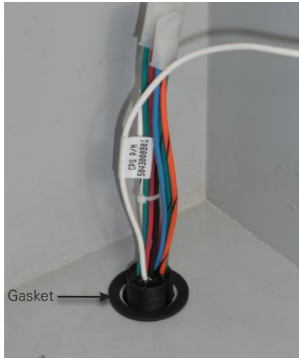
Figure 32. Pigtail internal gasket installation.
