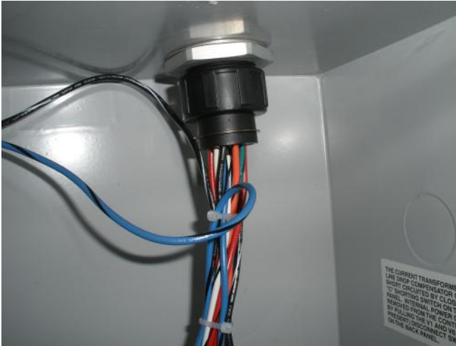
Figure 20. Installed pigtail connector on control cable.
