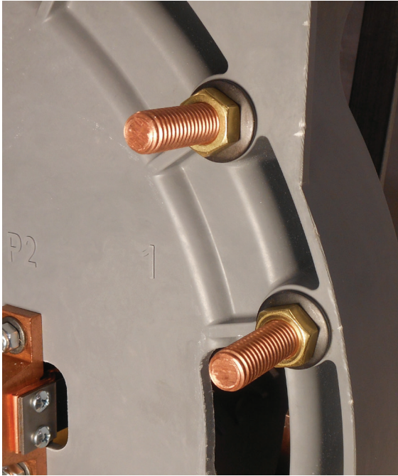
Figure 5. Main stationary contact hardware.
