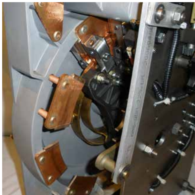
Figure 80. Stationary contact removal.
