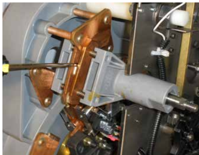
Figure 41. Positioning reversing movable contacts.
