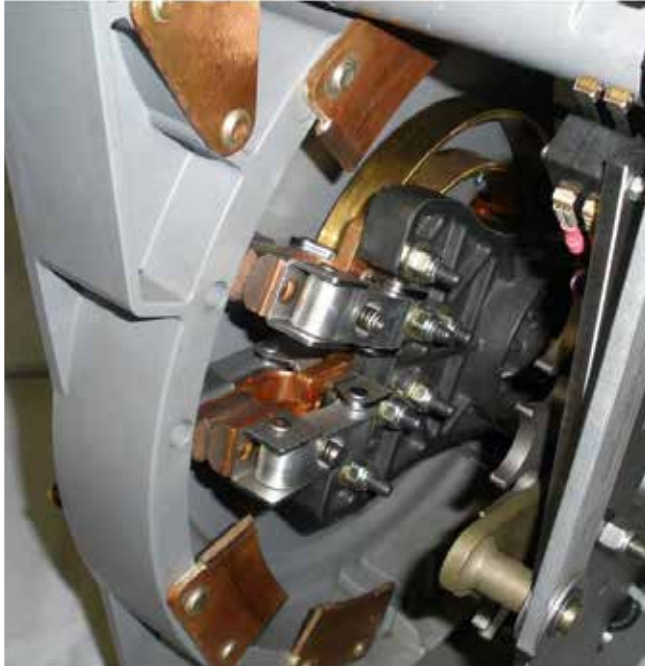
Figure 131. Main movable contacts in number 1 stationary position.
