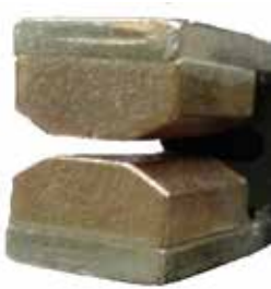
Figure 17. QD5 tap-changer movable contact.
