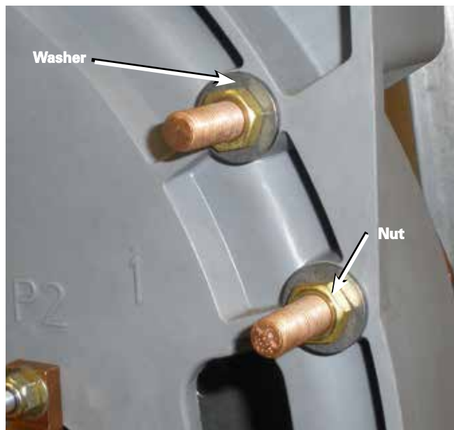
Figure 81. Contact hardware installation.
