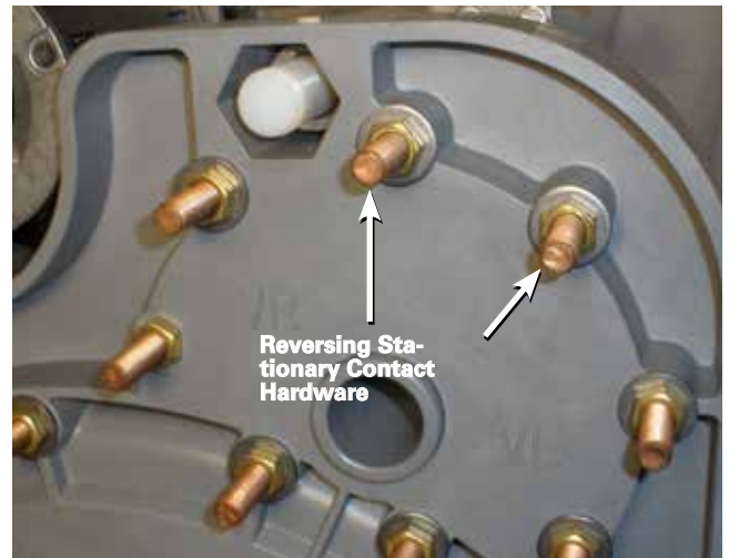
Figure 36. Reversing neutral stationary contact.
