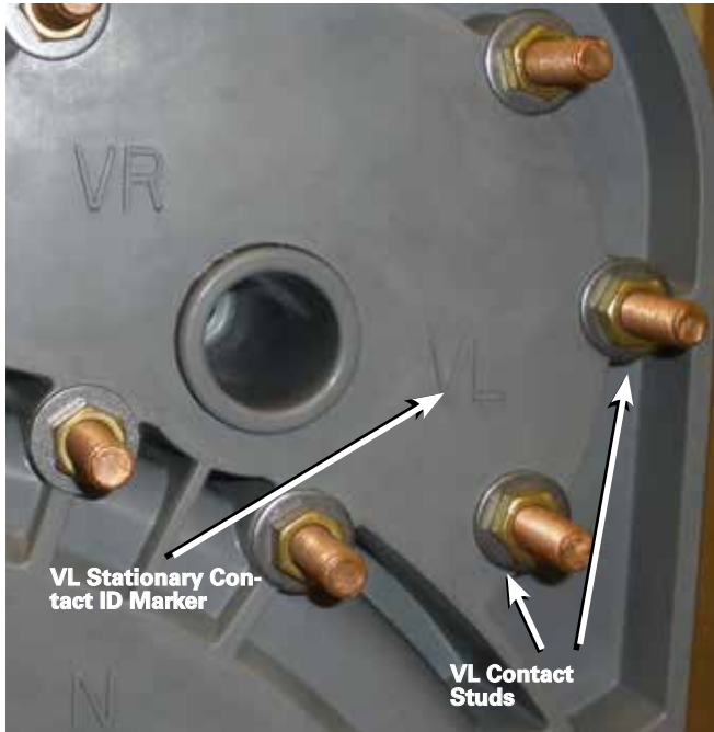
Figure 89. VL reversing stationary hardware and ID.
