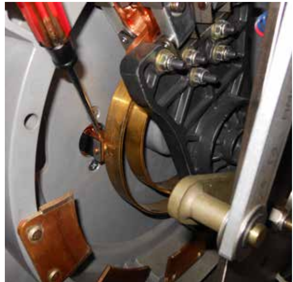
Figure 142. Inserting the outer contact ring between the button contacts.
