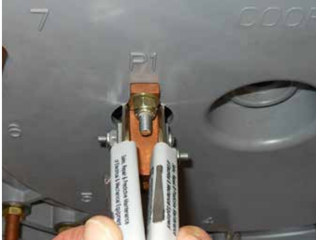
Figure 144. Installing ring into P1 contact.
