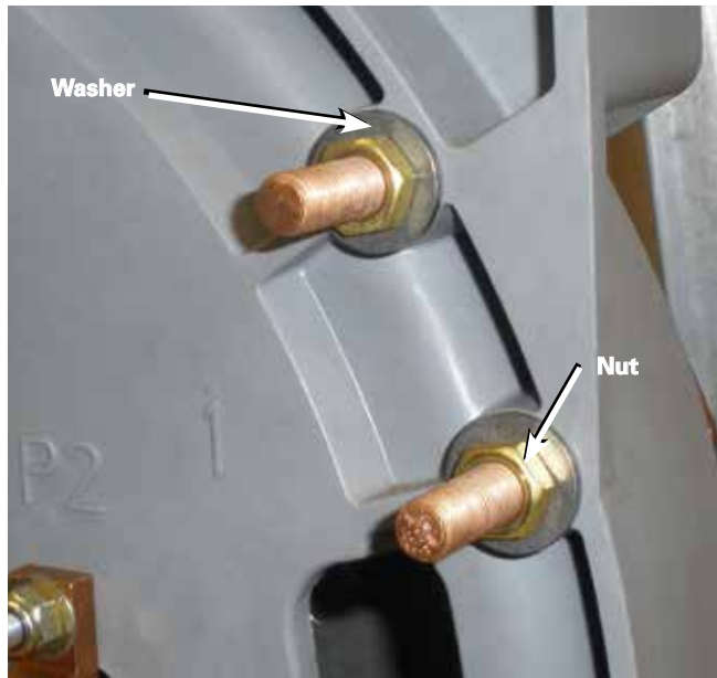
Figure 5. Contact hardware installation.
