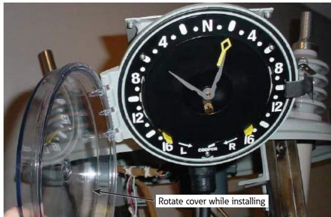
Figure 5. Main cover rotation during installation
