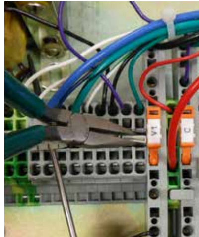
Figure 23. Removing jumper between C2 and C3.
