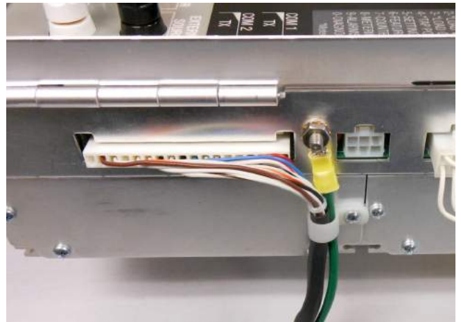
Figure 31. Installing ground wire and General Electric fork-style wiring harness
