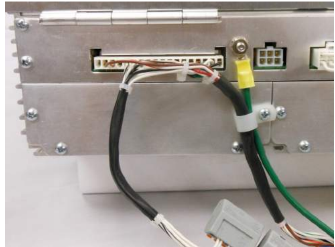
Figure 39. Installing ground wire and General Electric pin-style wiring harness
