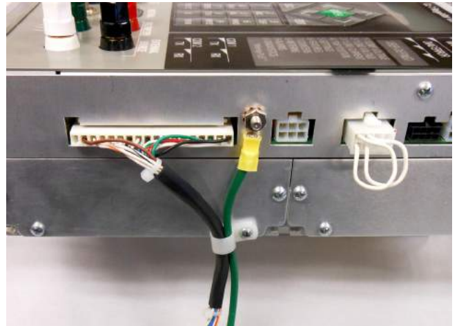
Figure 46. Installing ground wire and Howard Industries wiring harness
