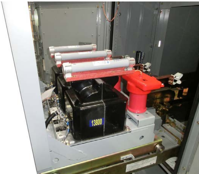
Figure 41. Typical VT Drawer Drawn Out onto Extension Rails.
