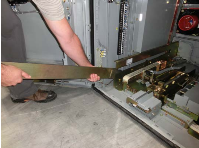
Figure 8A. Insertion of the Draw-out Extension Rails.
