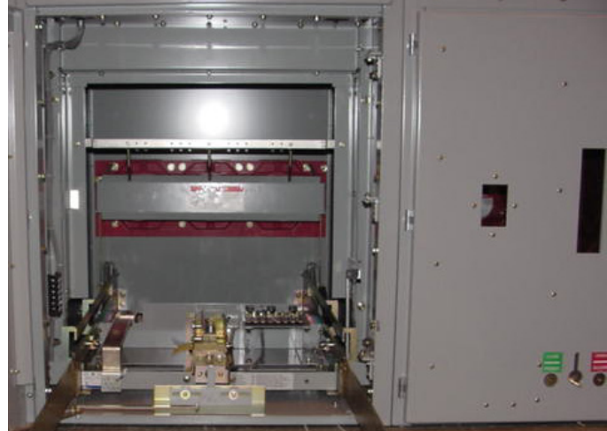
Figure 42. Typical Auxiliary Compartment (VT Compartment Shown with VT Drawer Removed).
