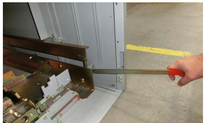
Figure 39. Hand Operation to Manually Open the Shutters.
