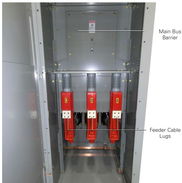
Figure 4. Removal of Necessary Barriers.
