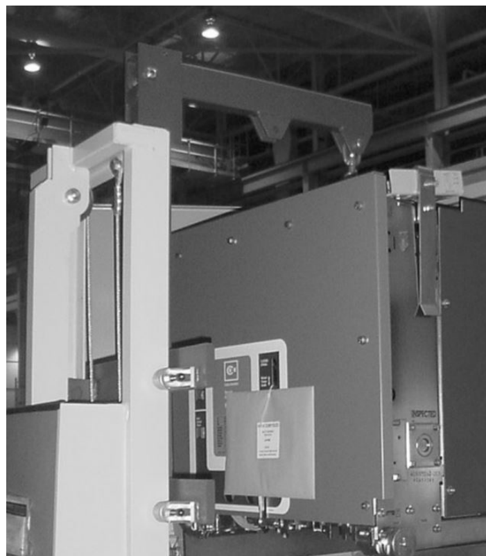
Figure 3. Lifting and Setting the Breaker in the Housing.
