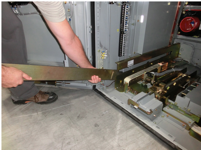
Figure 2. Insertion of the Draw-out Extension Rails.
