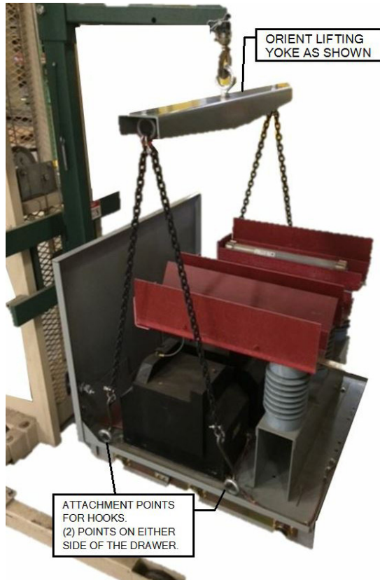
Figure 4. Lifting and Setting the Auxiliary onto the Extension Rails.
