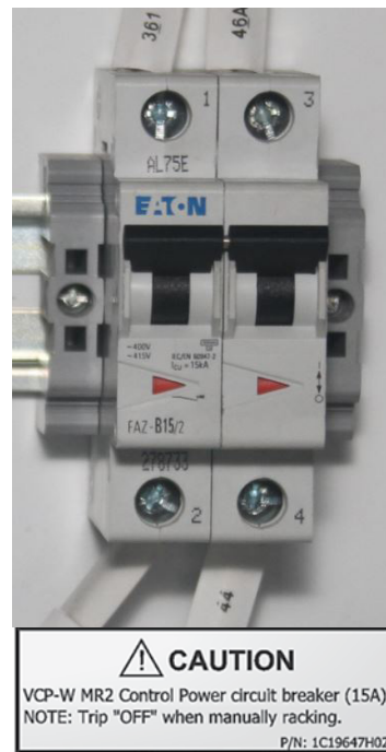
Figure 11. 15 A circuit breaker.
