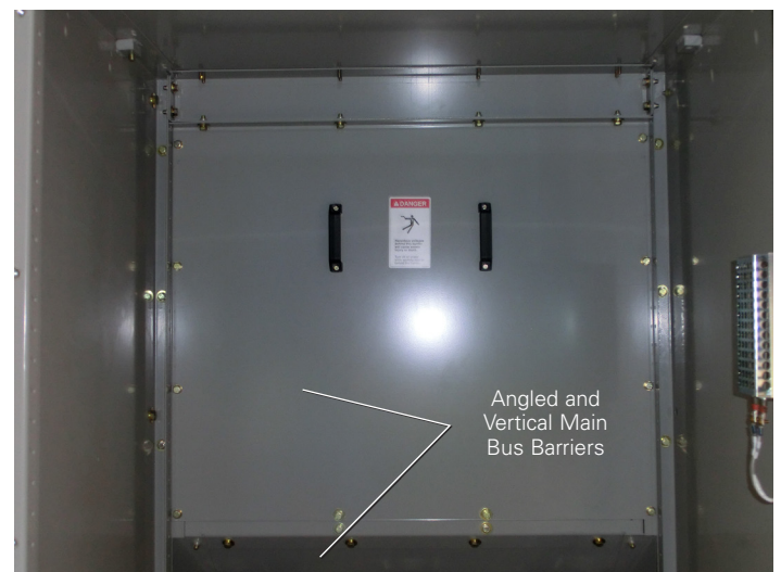
Figure 3. Main Bus Installation – Bus Barriers Shown.
