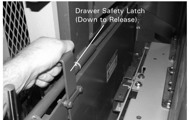
Figure 29. Releasing the Transformer Drawer from the Lifting Pan.
