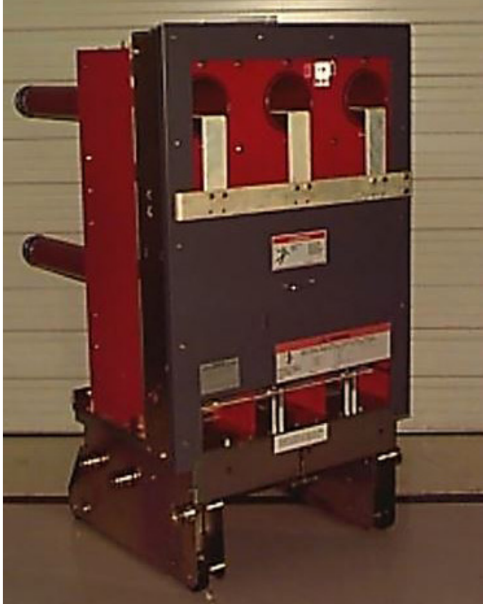
Figure 32. Manual Ground and Test Device.
