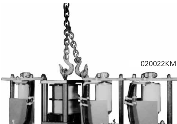
Figure 25. Lifting mechanism in and out of recloser head
