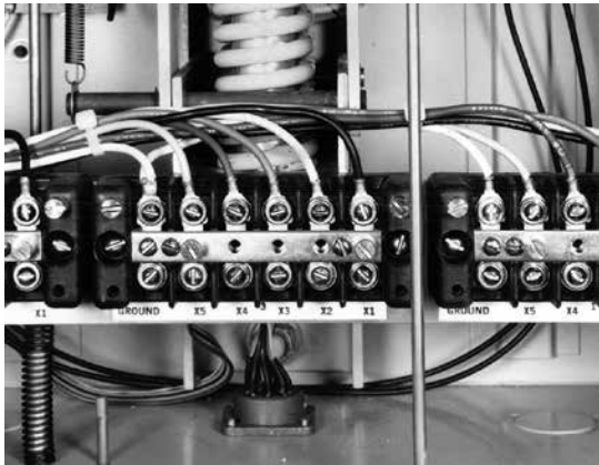
Figure 6. Position of shorting thumbscrews (as shipped)
