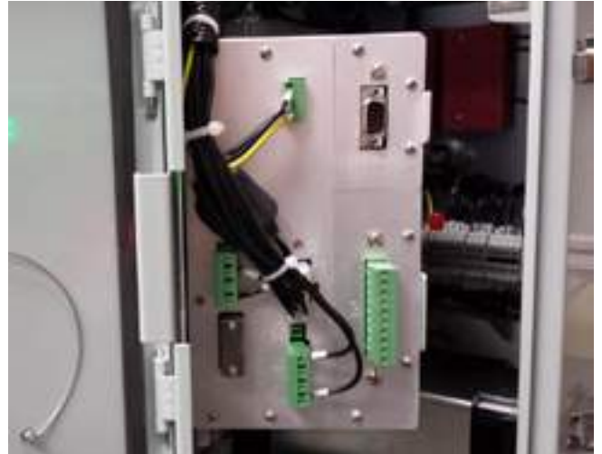
Figure 38. Side swing-panel view of SPEAR single-phase recloser control
