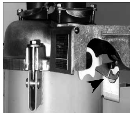
Figure 1. The non-reclosing feature is set with a handle under the sleet hood (see arrow). When the handle is down (top), the recloser will trip on overcurrent and lock out without reclosing. When the handle is up (bottom), the recloser will operate according to its internally set program.
