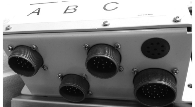
Figure 2. Disconnect the cable(s) at the recloser and junction box
